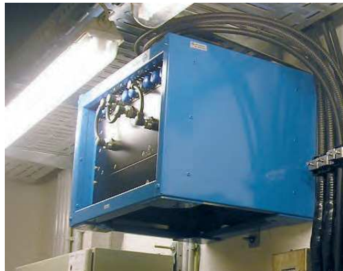
MNCS®-Schrank im Innenbereich MNCS® rack as compact wall-mounted solution
