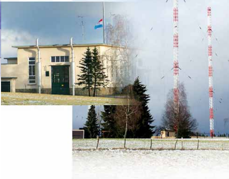
Broadcasting Center Europe Station (BCE) in Marnach
